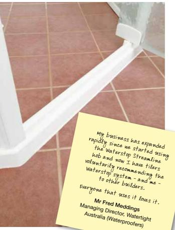
This is by far the easiest way for building and construction companies to comply with the revised Australian Standard in waterproofing (AS 3740-2004), which requires a water barrier with a minimum of 5mm above the finished tile line. The product is colour finished and does not require covering or capping.
